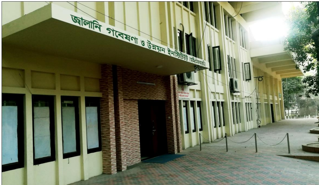
Institute of Fuel Research and Development (IFRD) Building
