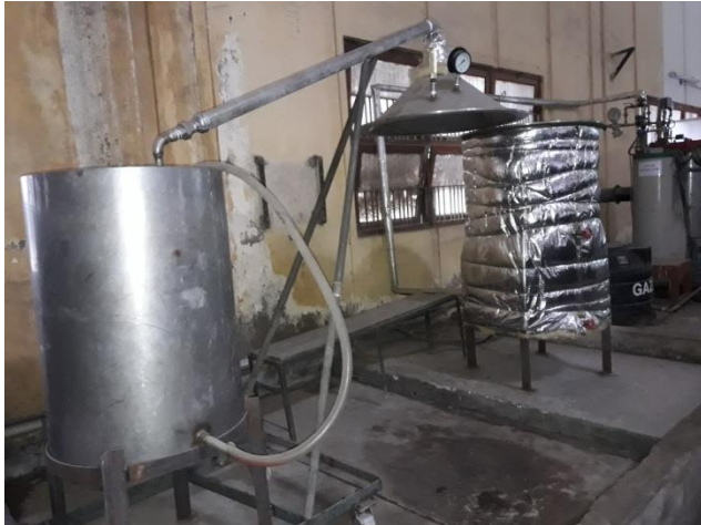
Steam distillation pilot plant
